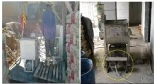
Figure 2 - In-site made "steps" for working process improvement
