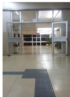
Tactile floor does not embrace the main of the university (Authors' photo)
