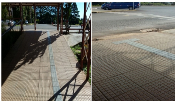
Front ramps of the university access (Authors' photo)
