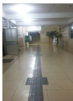
Tactile floor in the university corridors locations (Authors' photo)
